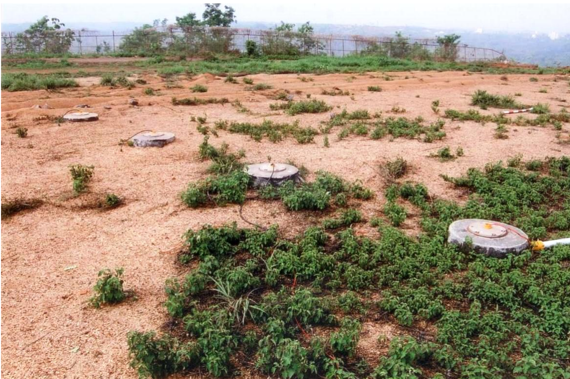
Photo 30: RESA for R/W 24 at Mangalore on the Day of Accident
