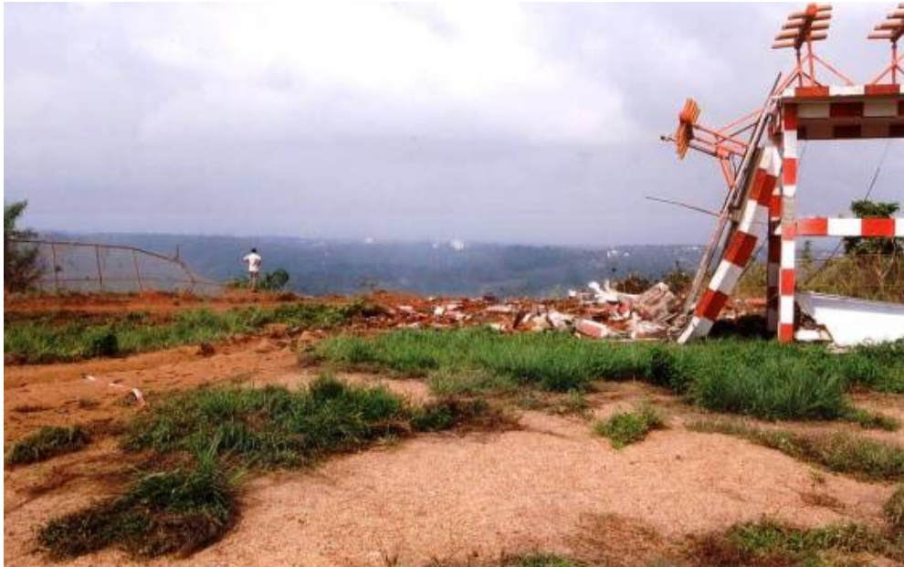
Photo 9: Broken ILS Mounting Structure Due to Impact of Wing
